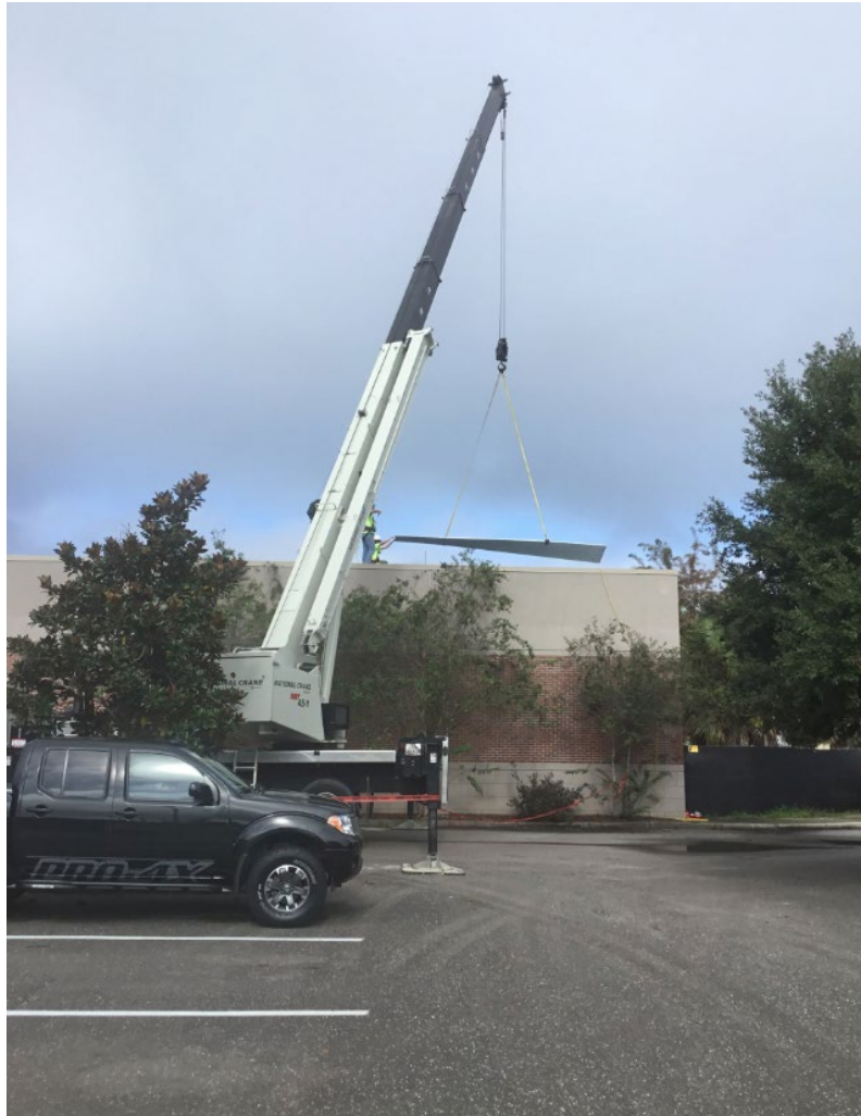
Steel Grate Removals from Equipment Yard for Chiller #4
